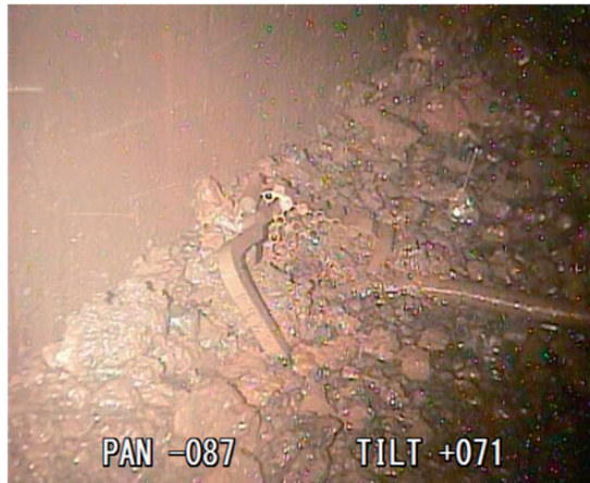
Fig. 4. Inside the bottom of the primary containment vessel, adjacent to the inner wall of the pedestal, in Unit 2.
